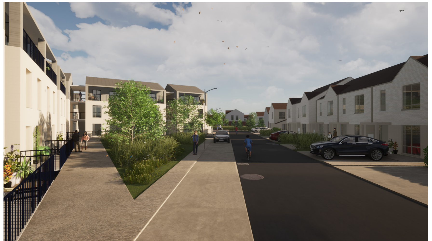
View of duplex apartments and terraced houses overlooking common public space
