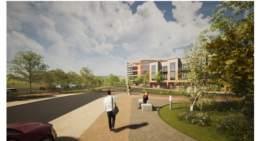
Street View looking North to landmark 5 storey building on Lissywollen Avenue/ Brawney Road
