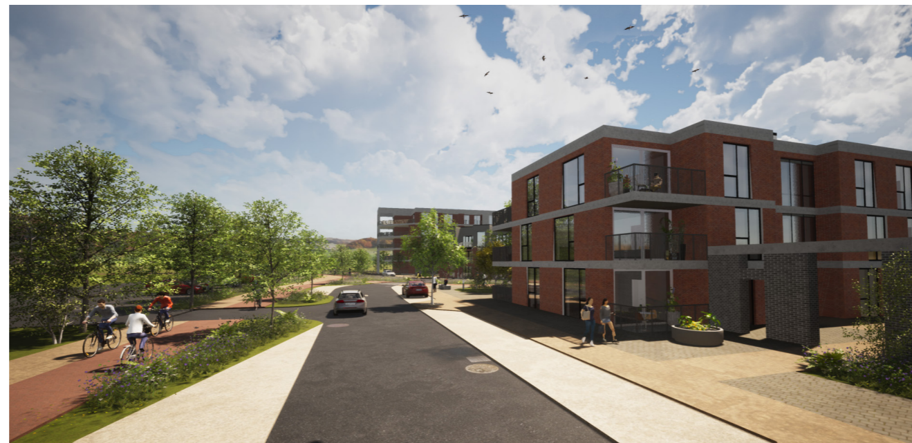
Street View looking north to Block P, with the cycle track and Gaelscoil to the left
